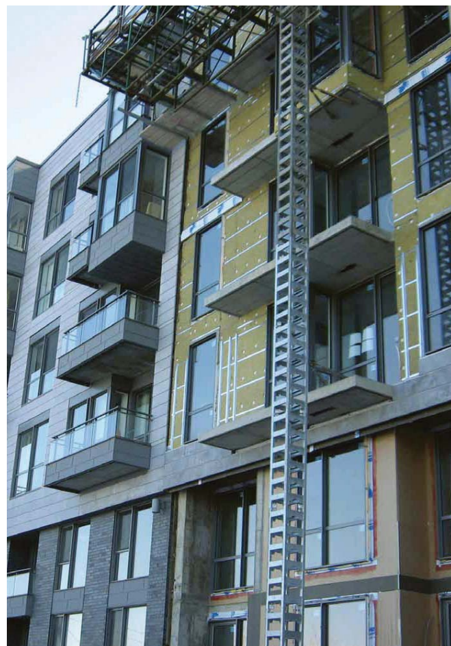
Soleno Project, Montreal PQ Roxul CavityRock® MD
